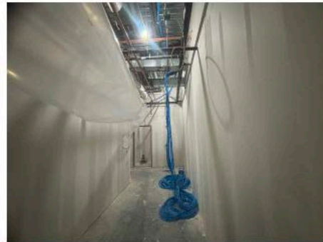
Security & network cabling being installed
