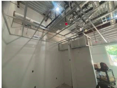
Ceiling grids and light fixtures being installed
