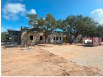
Entry from parking lot
