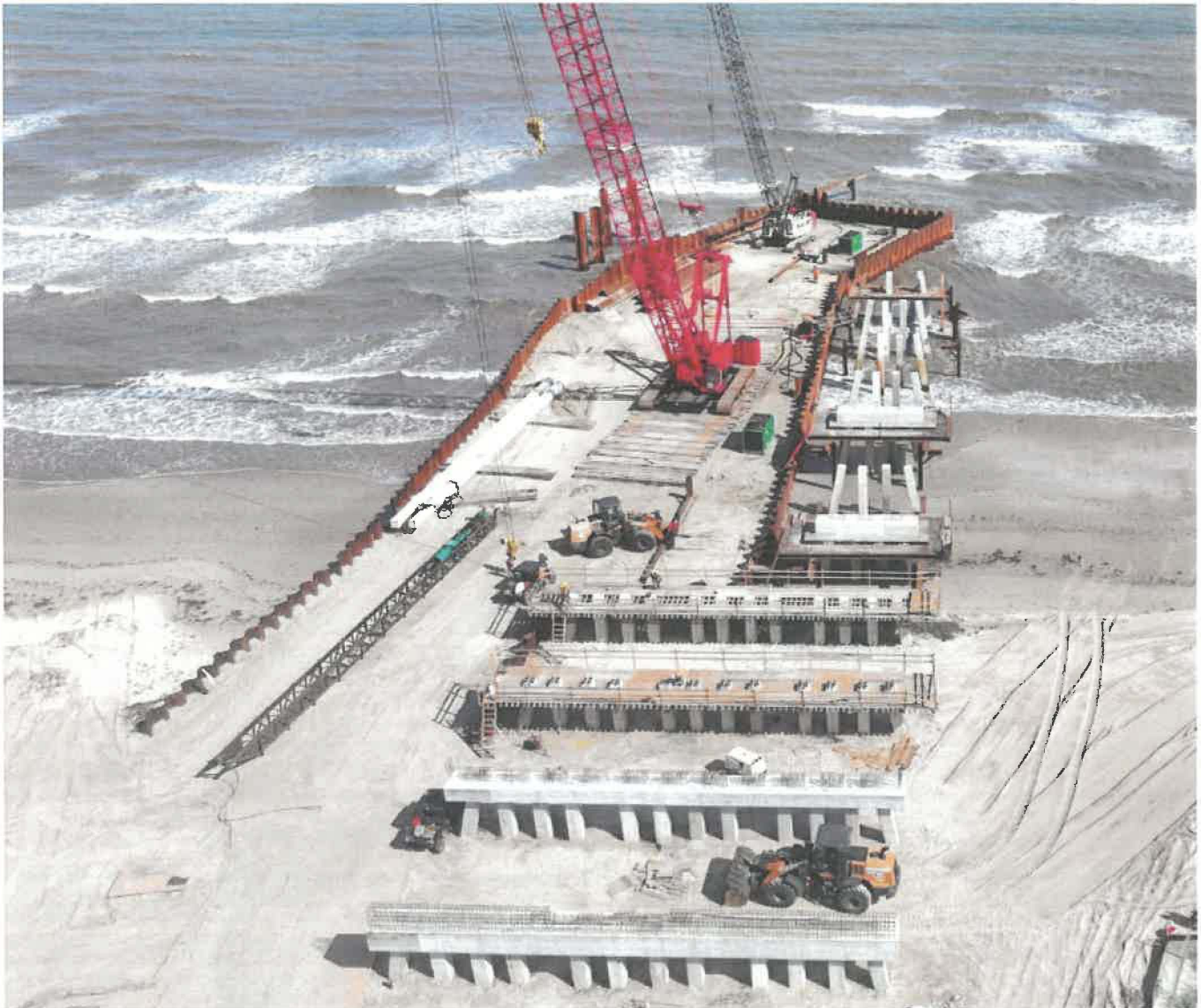
Rollover Fishing Pier Construction Progress
