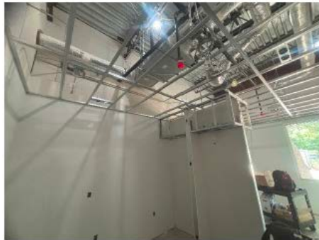
Ceiling grids and light fixtures being installed
