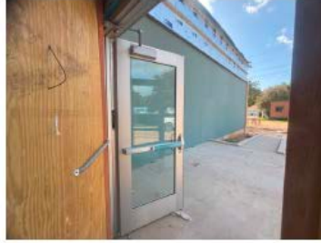
Doors have been installed
