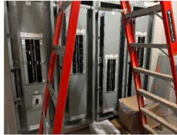
Electrical panels being installed
