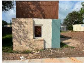
Mock wall approved by architect
