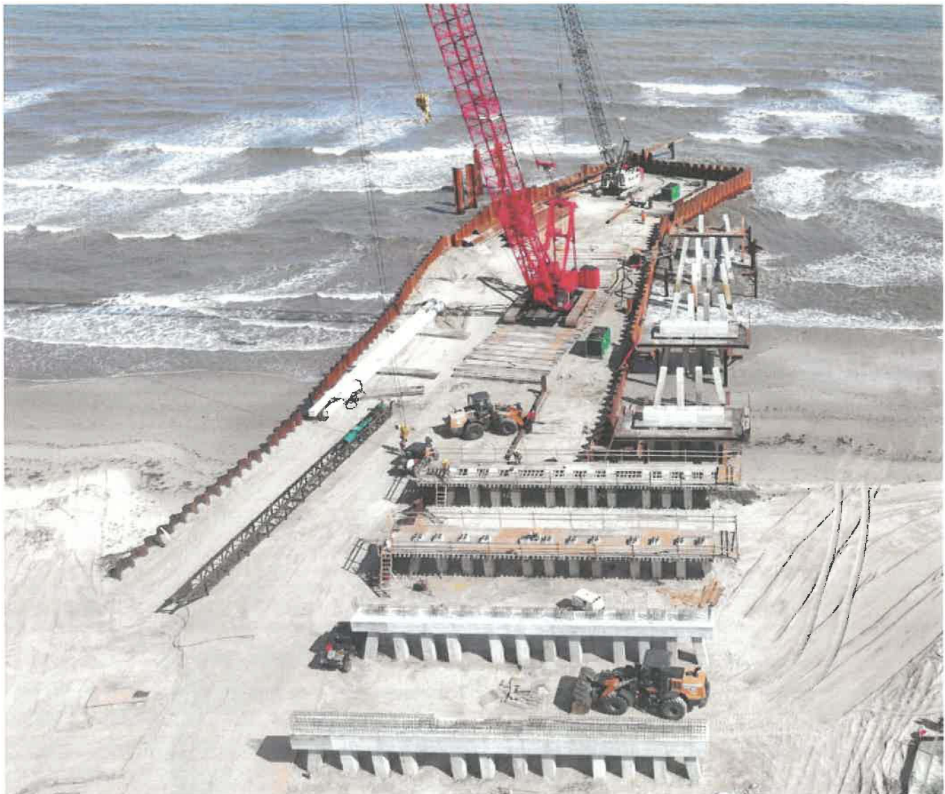
Rollover Fishing Pier Construction Progress
